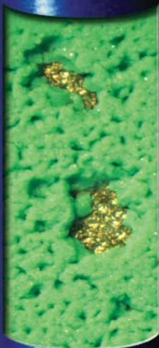
Cavitation erosion Scotchkote® epoxy
